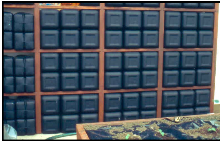
Milk jug water storage wall in a passive solar hobby greenhouse – Disposable milk jugs on left and returnable milk jugs on right are spray painted flat black. In this well-built structure, nighttime temperatures dropped to 39° with no supplemental heat when outside temperatures dropped to –17°.
